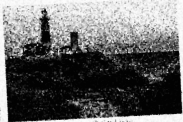
Montauk Point Lighthouse
